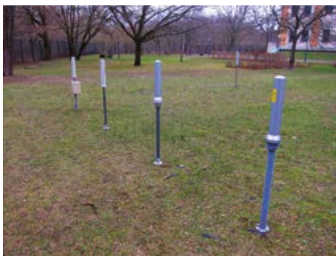
Test probes at the BFS premises in Berlin, showing antennas in various stages of development. Each can be equipped with a pair of Geiger-Muller counters, one for low and one for high dose rate. Source: Peter Bossew.
