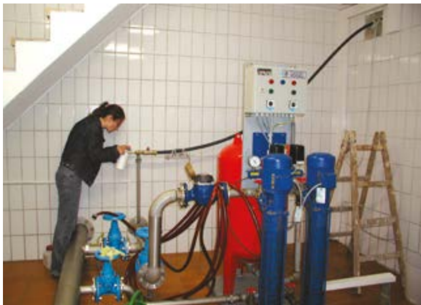
Water sampling in a pump house of a waterworks, Austria. Source: Valeria Gruber.
